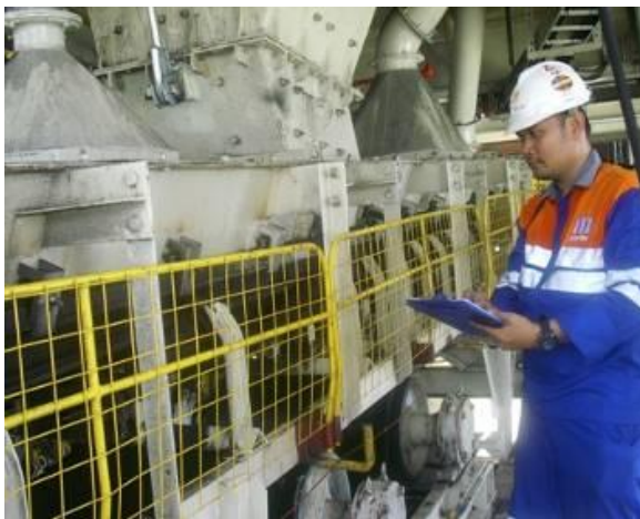
Figure 4. Assessment of coal handling facility by consultant
