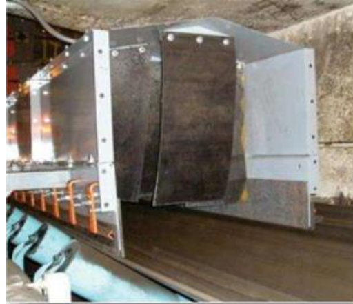
Figure 9. Rubber curtain inside the chute
