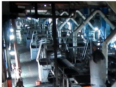
b. After Improvement (dust free) Figure 13. Coal dust at belt conveyor – coal bunker area
