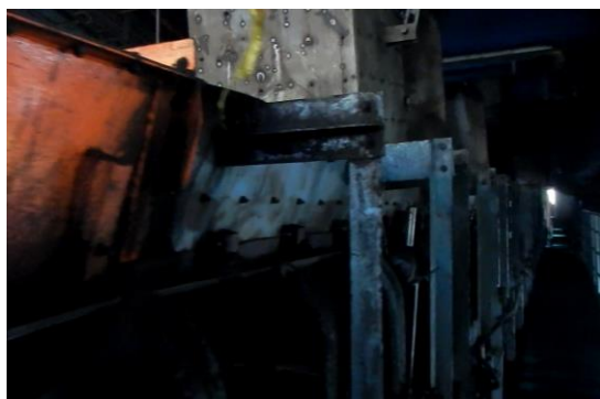
b. After Improvement (dust free) Figure 12. Coal dust at belt conveyor - transfer point area
