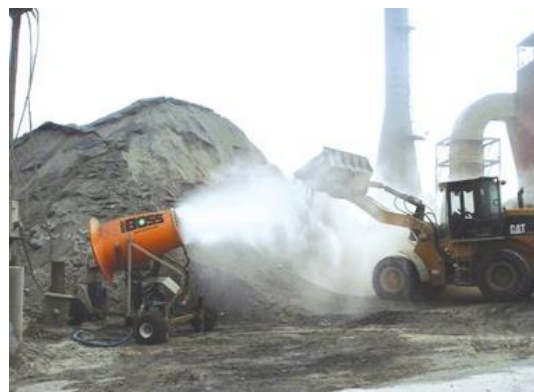
Figure 11. Dust boost at stock pile area
