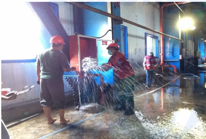
Kebocoran Valve di Belt Conveyor
