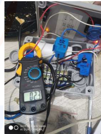
Figure 6. Testing of SCT013 sensor
