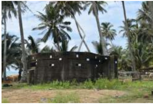
Figure 12: The structure and surrounding area of the pillbox at Kg Anak Rhu, Bachok, Kelantan. Source: Field study.
