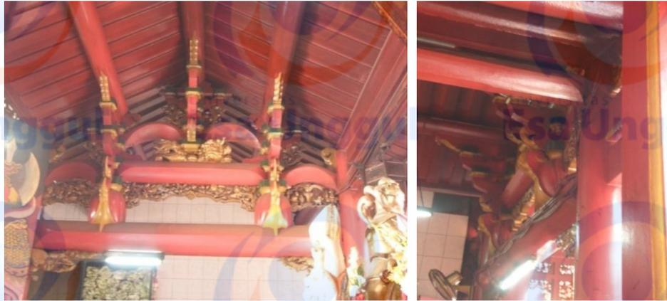
**Gambar 18. Rangka Penahan Atap Kelenteng Bagian Depan**
