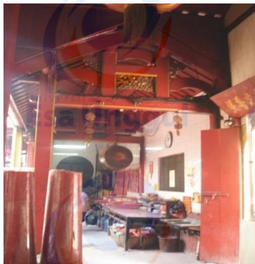
**Gambar 19. Rangka Penahan Atap Kelenteng Bagian Tengah**
