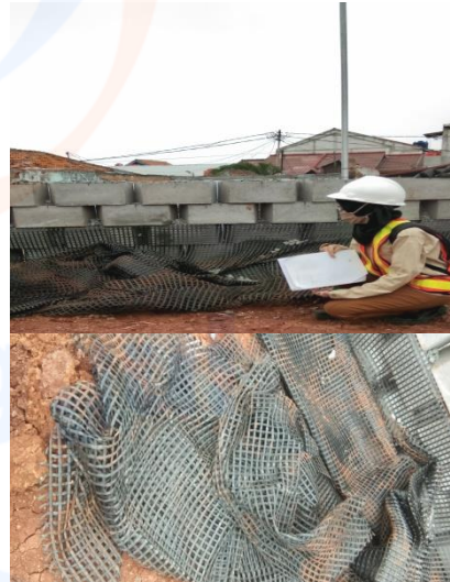
SRW Sregmantal Retaining Wall
