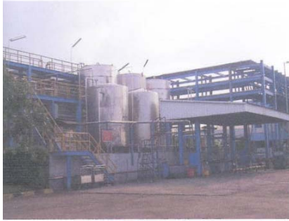
Oil Storage Tank
